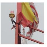
The ABC-7L Weatherproof Obstruction Light is specially designed for a wide variety of cranes used in harbours, metallurgies, mines, lighthouses and tall buildings. It consists of LM6 die cast aluminium base and high-intensive glass (or PMMA material), which houses the electronics and LED bulb, providing environmental protection and shockproof. The application in harbours shows its perfect waterproof and corrosion resistant performance.
